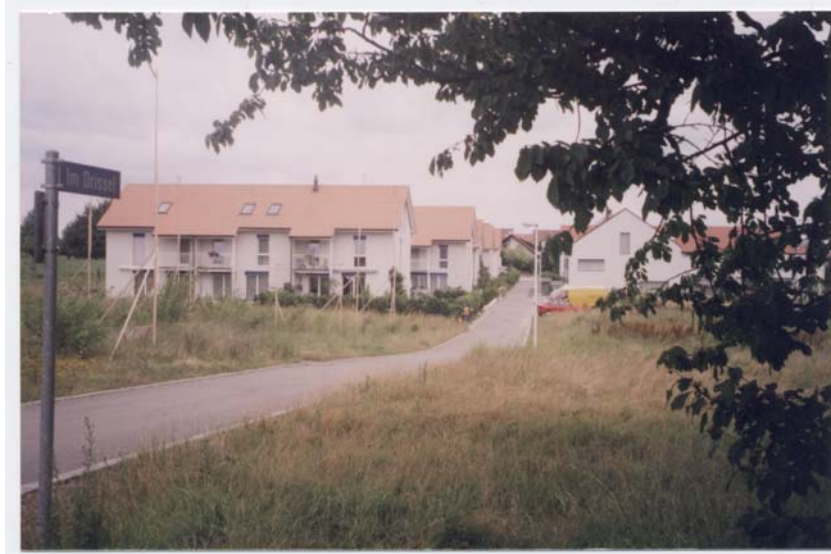
A neighborhood of 80 townhouses at Basel (Switzerland) constructed in CLC density 1400 kg/m 3
