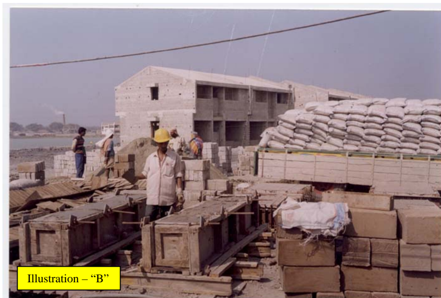
CLC block masonry density 1,400 kg/cum used for Colony near Calcutta
