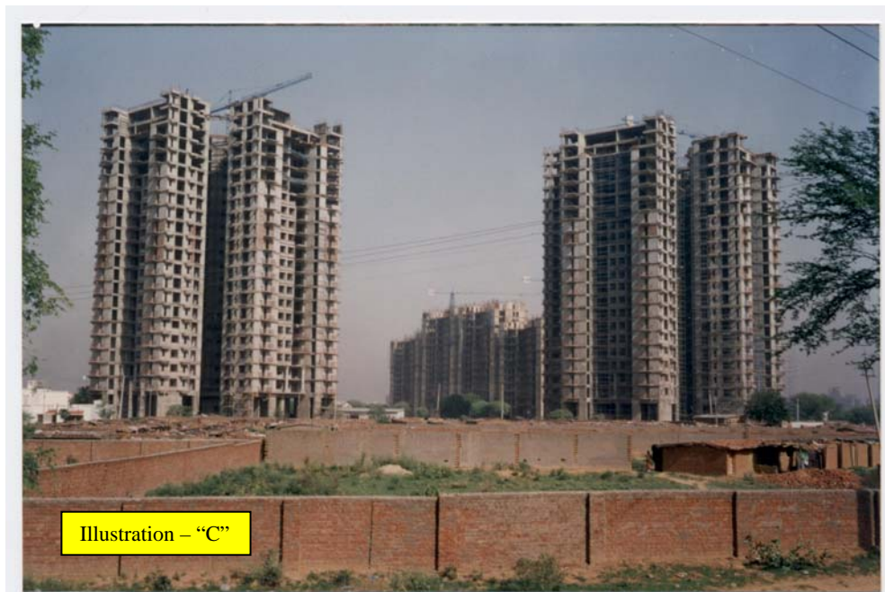
CLC blocks of density 1000 kg/cum used in such towers south of New Delhi
