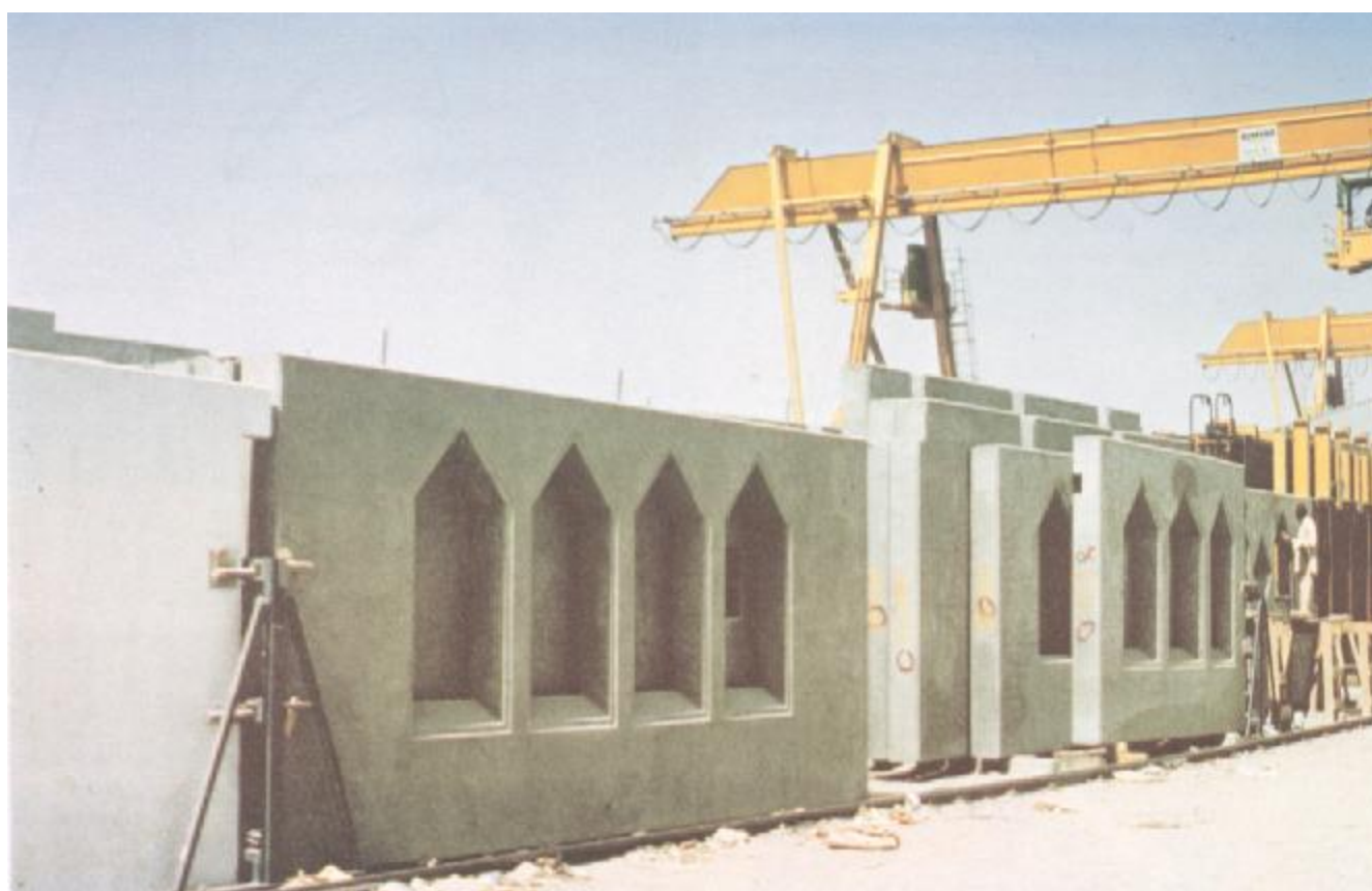
Vertically cast panels for government agriculture schools in Middle East, density 1400 kg/m 3
